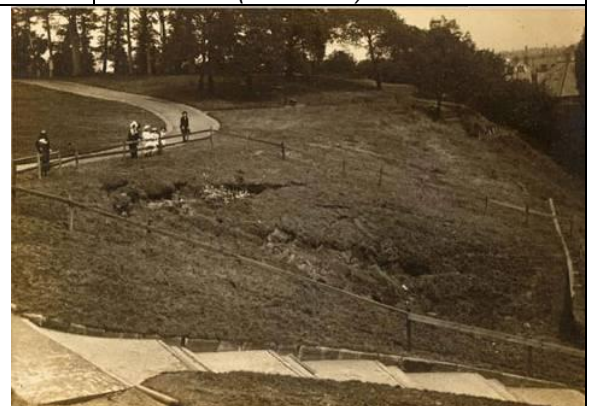
17. Collapse adjacent to steps in the park, possibly the same area as 16.
