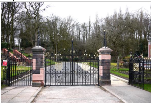
38. Restored gates and gate piers
