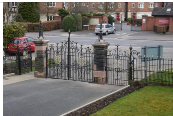
39. Restored gates and gate piers
