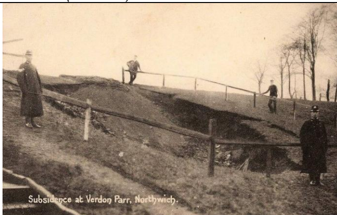
16. Subsidence on the slopes of Verdin Park
